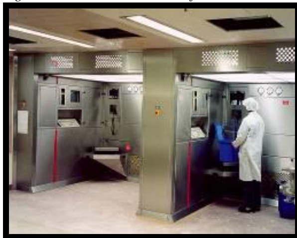
Figure 3.9.4 Downward laminar flow booth
